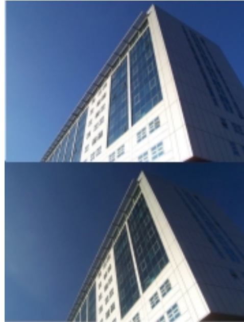
By turning the polariser's outer ring you can make colours richer and reduce reflections. In this architectural photo adding the filter makes the sky more blue and reflections are reduced.
