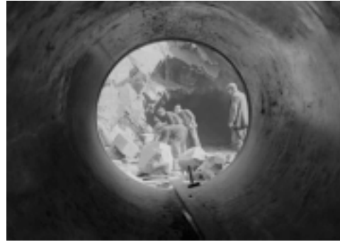
The tube is an effective means of drawing the viewer's eye onto the workers.
