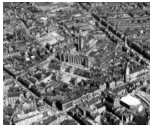
The view from the sky makes the town look small. It is a good use of scale.
